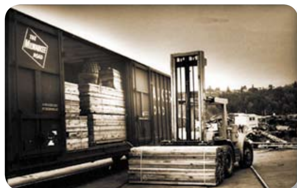
Railcar Loading Operation - undated
